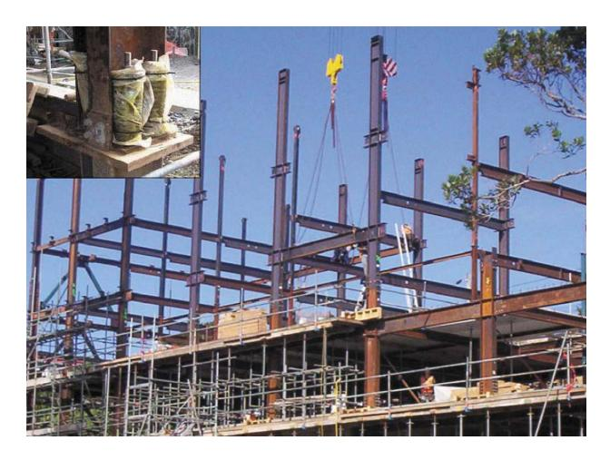
Figure 7 Aurecon's International Structural Engineers UK award winning Te Puni student accommodation project which incorporates damage-avoidance rocking frames (inset) and sliding hinges – both developed via Heavy engineering industry levy funded research and government funding.
