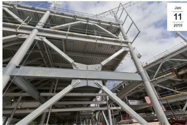
The Regional Science and Innovation Centre (RSIC). Here the steel construction allows a structure with open spaces and free circulation to enhance the collaboration process. The main seismic resisting elements are the Buckling Restrained Braces (BRB) manufactured by our members D&H Steel under license from Star Seismic.
